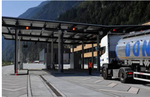
Figure 6 - Ripshausen HGV control centre
