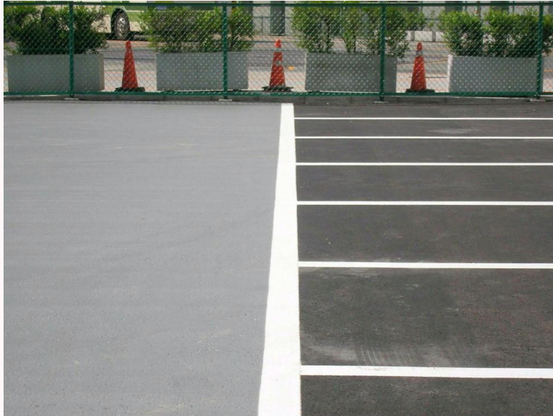
Solar Heat-blocking Pavement
