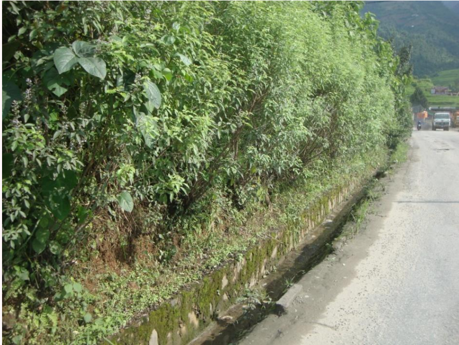
Line of Palisades keeping side drain clean, Naubise – Thankot Road, Nepal
