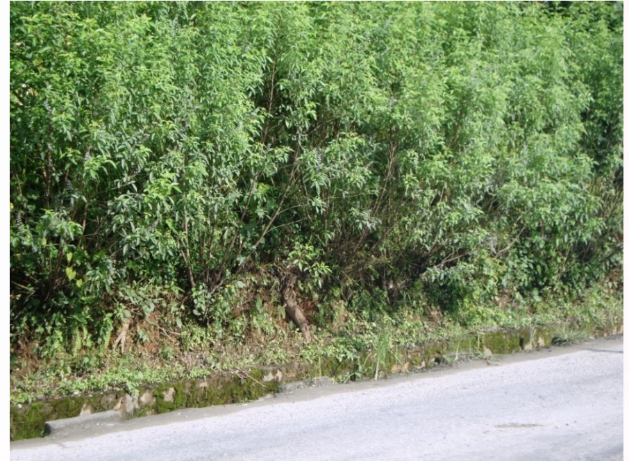
Line of Palisades keeping side drain clean, Naubise – Thankot Road, Nepal
