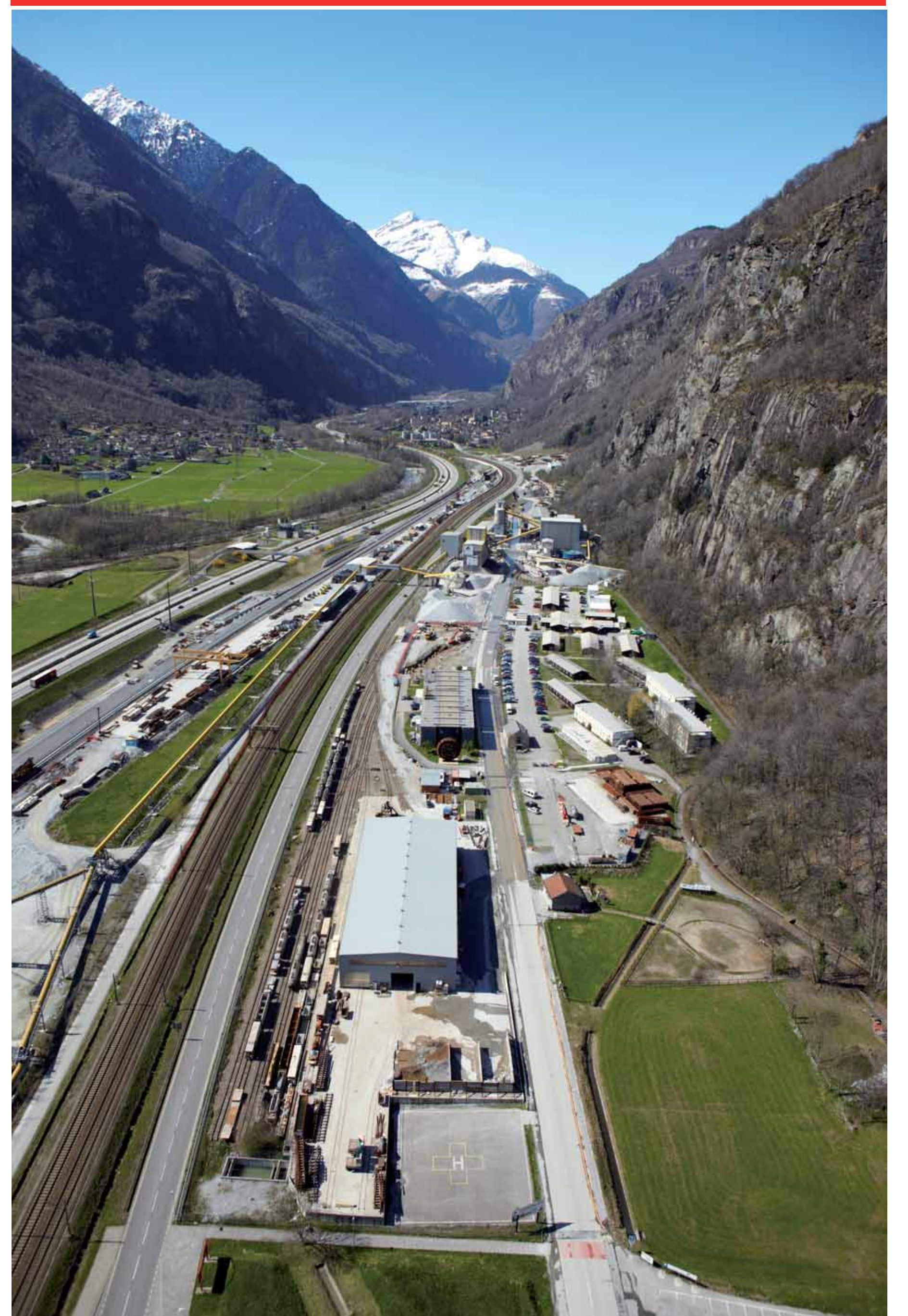
The Saint-Gotthard range makes for a natural barrier between northern and southern Europe. This shot was taken near the southern entrance to the rail tunnel. © Alp Transit Gotthard AG
