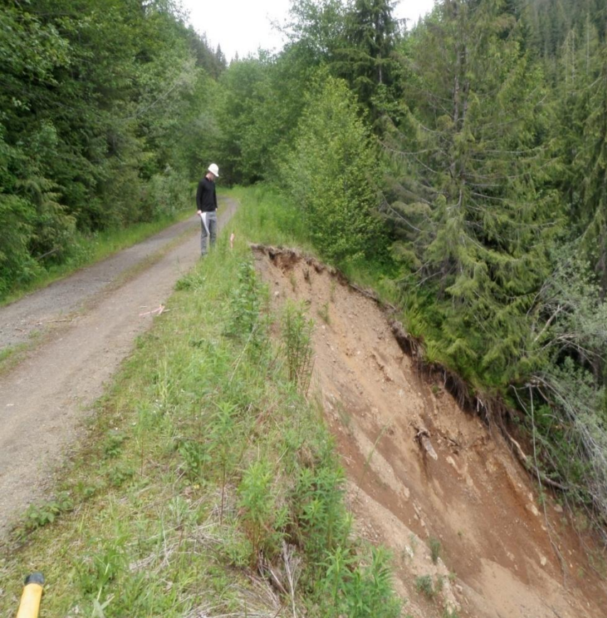
TYPICAL VIEW OF A SIDECAST FILL PRIOR TO FAILURE
