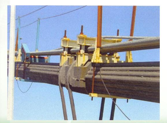
Installation of auxillary suspension (4 x 19T15 stands
