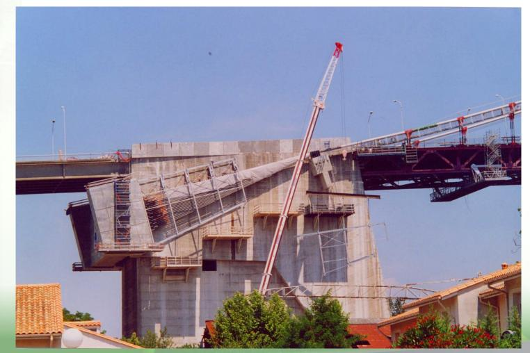
Air tight covering of the anchoring chambers
