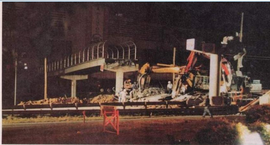
Contractors demolishing the remaining sections of the failed bridge.
