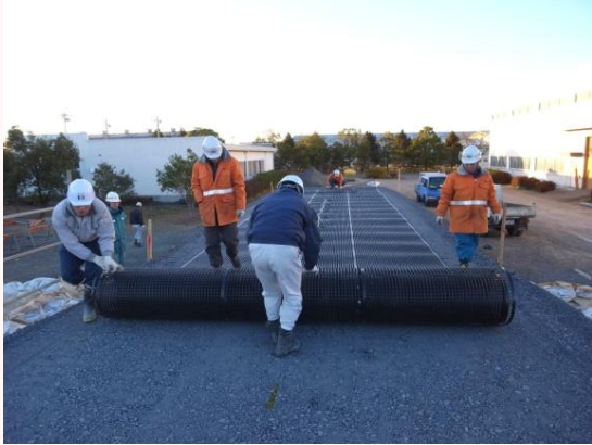
1) Geosynthetics placement
