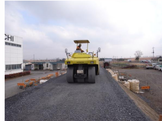
1) Compacted crushed stone
