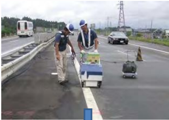
Cavity research by GPR
