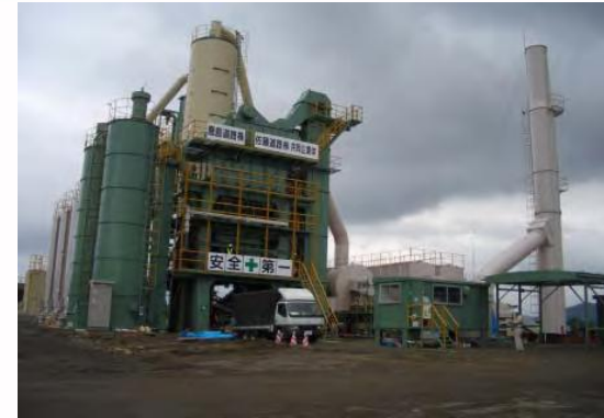
Temporary asphalt plant
