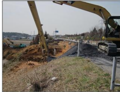
3/14 11:00 Removing collapsed embankment
