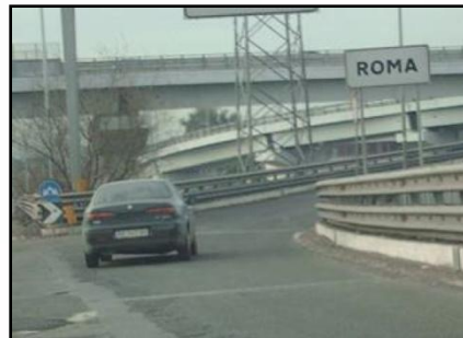
PAVEMENT MARKING NOT PRESENT
