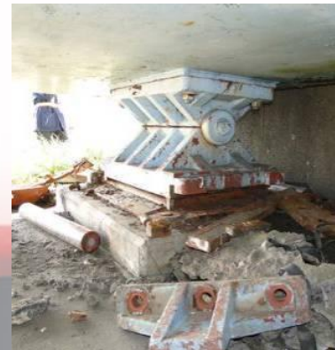
Damage to movable bearing
