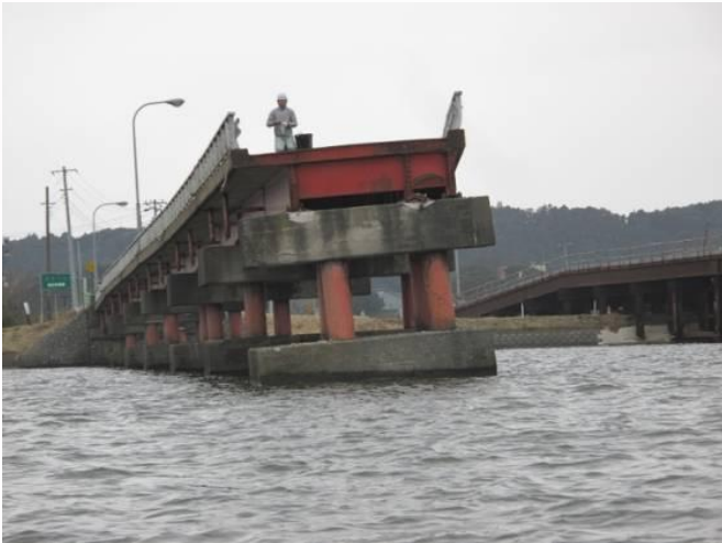
Collapse of bridge with pile-bent columns
