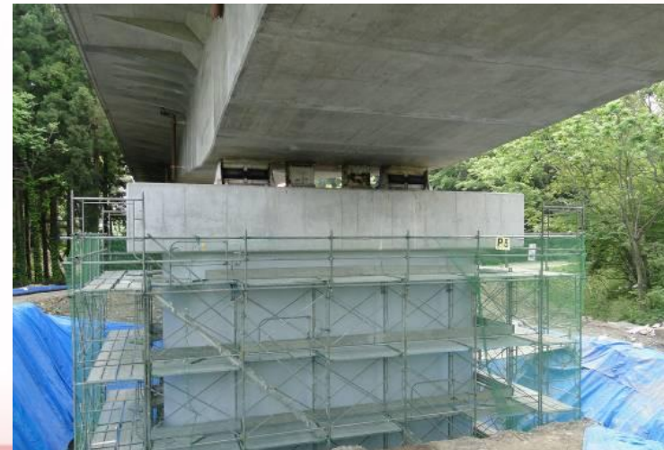
Temporary repair by wrapping up with carbon fiber sheet
