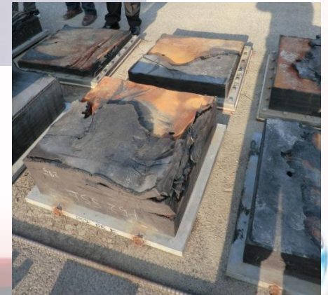
Ruptured rubber bearings
