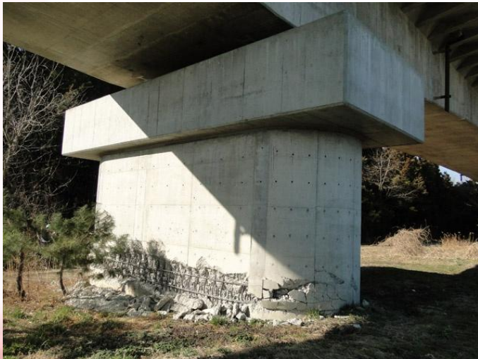
Damage to RC columns at section of cut-off of longitudinal rebars
