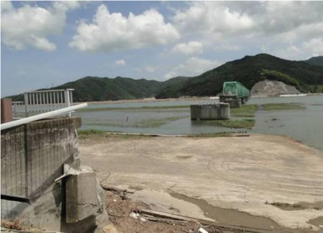
Shi-Kitakami Ohashi Bridge
