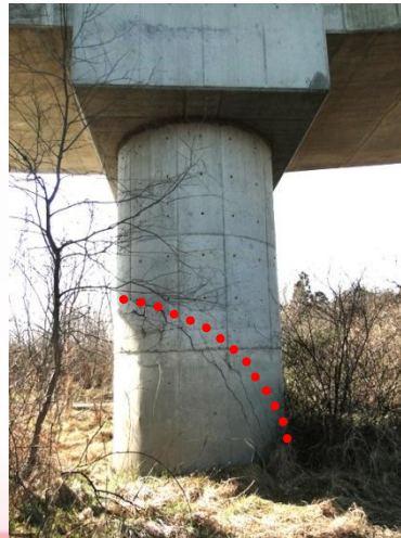
Damage to RC columns at section of cut-off of longitudinal rebars
