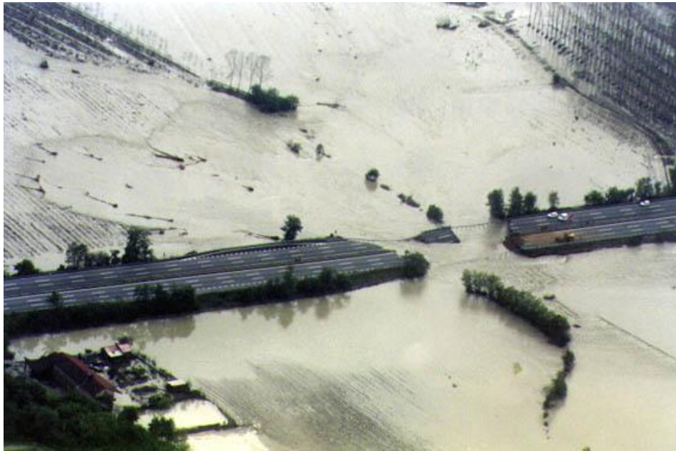
Flood 2000 on motorway A4 Northern Italy
