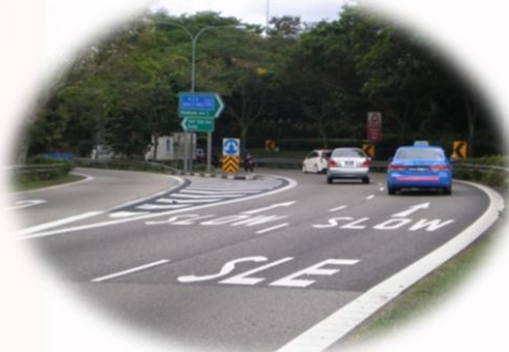
Resurfacing roads with high skid-resistance materials
