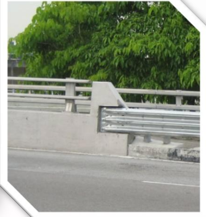
Provided proper transition of guardrail to parapet wall
