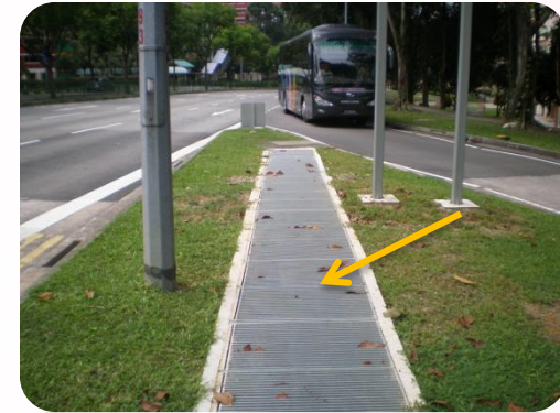
Covered drains to eliminate hazards
