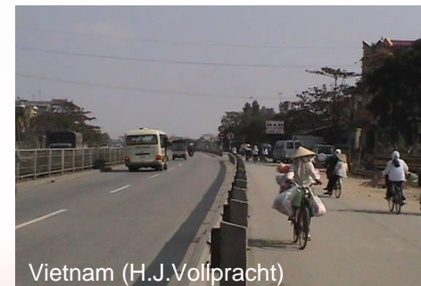
B - Pedestrian-bicycle path separated by narrow strip
