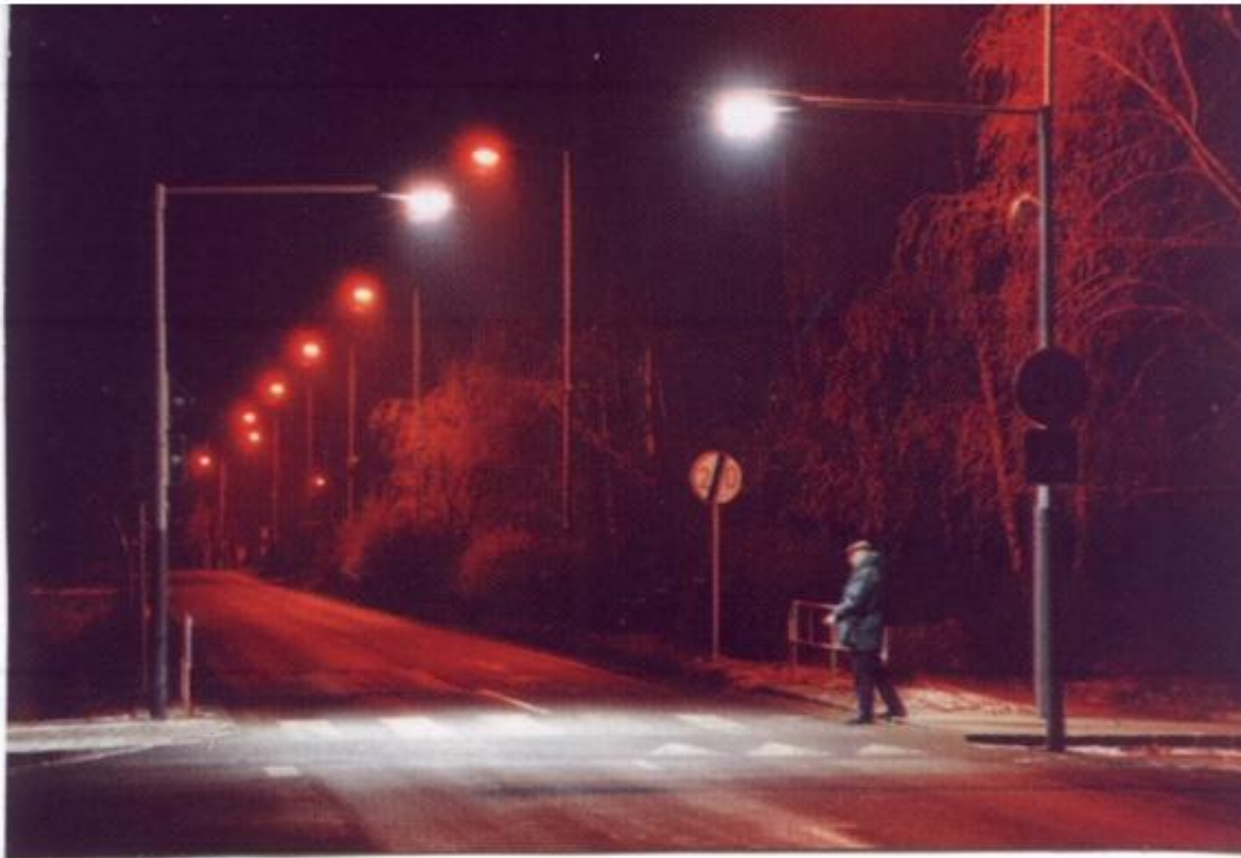
Additional traffic lights at the pedestrian crossing! (Photo pp1k_ing, Vladimir Mensik)
