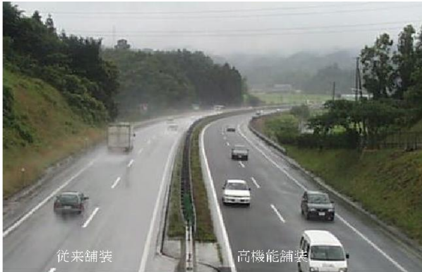
Old type pavement High Performance Pavement
