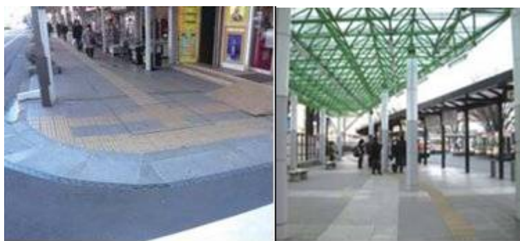
Figure 8 - Elimination of level differences on sidewalk,
