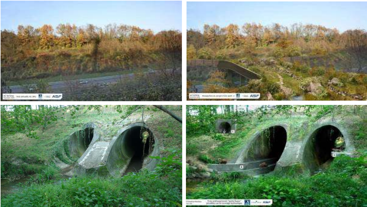
Figure 9 – Views of an ecoduct over the A7 (top) and of possible upgrades to a hydraulic structure on the A10 (bottom)
