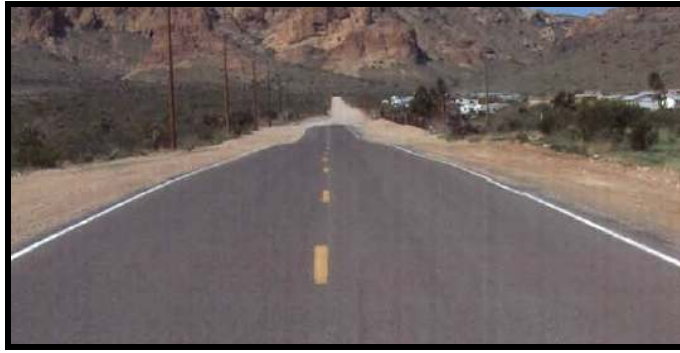
Figure 1 – Chip Sealed Road over Stabilized Subgrade
