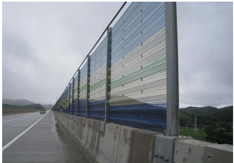
(b) Operation on bridges
