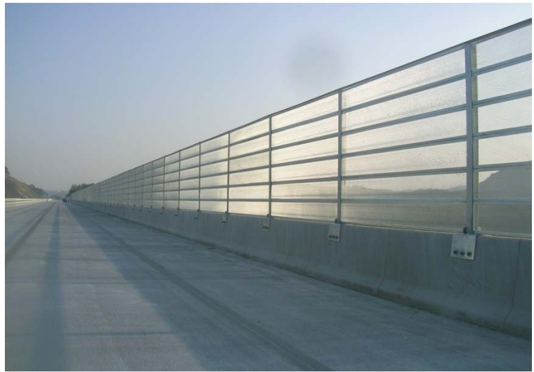
(b) Operation on bridges
