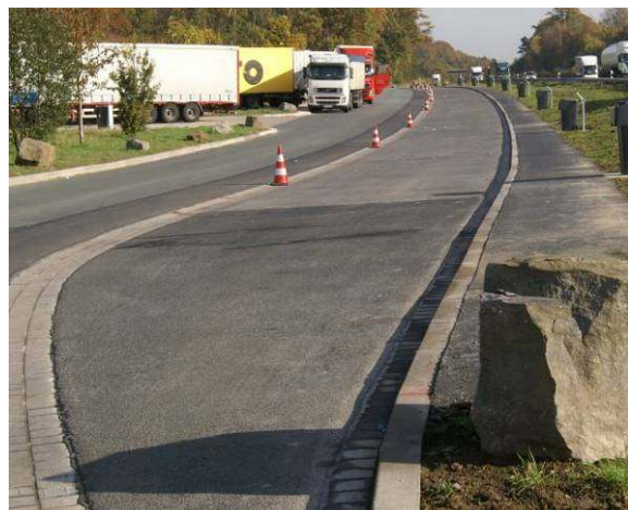
Figure 7 – View on the test road, parking-lot Highway A2
