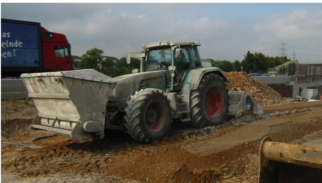
Figure 5 – Production of the soil-binder mixture for soil improvement
