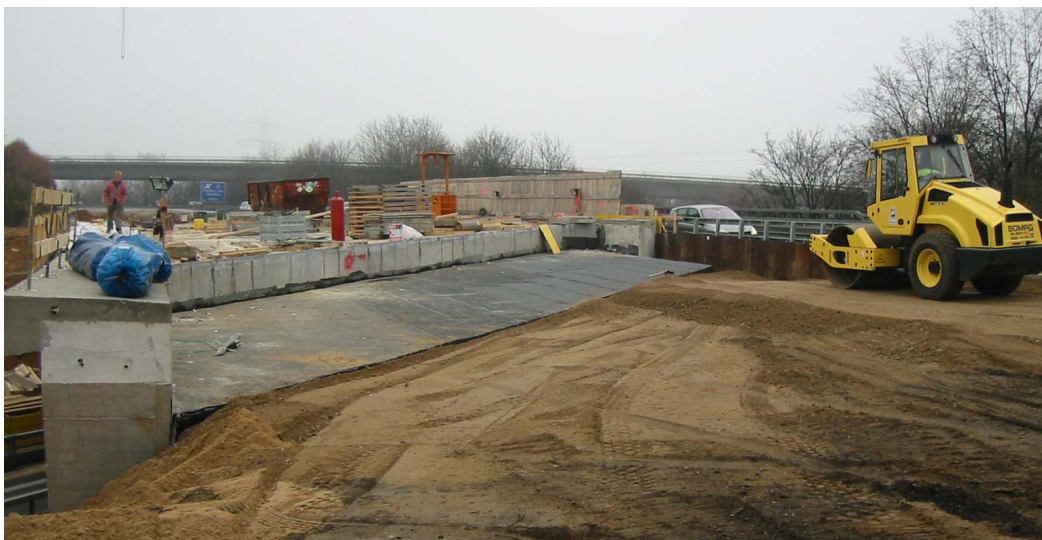
Figure 4 – Buried approach slab at backfill area 2
