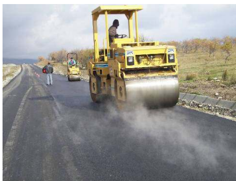
Figure 4 – Compaction equipment
