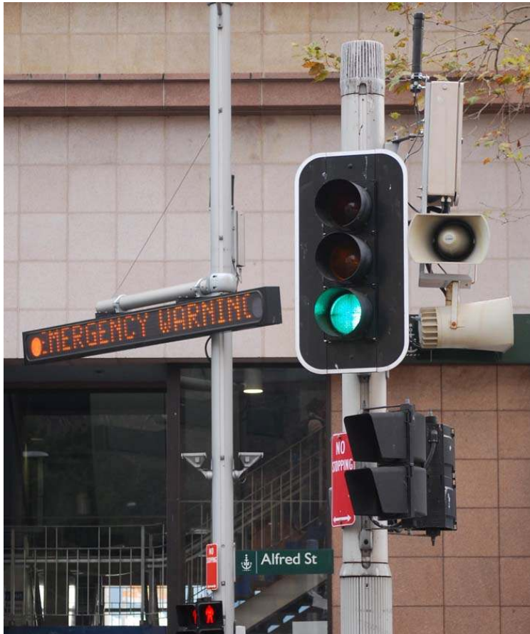
Figure 11 - Circular Quay VMS/radio and speakers/radio
