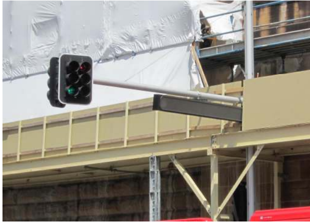
Figure 6 - George Street construction, safety barriers/scaffolding
