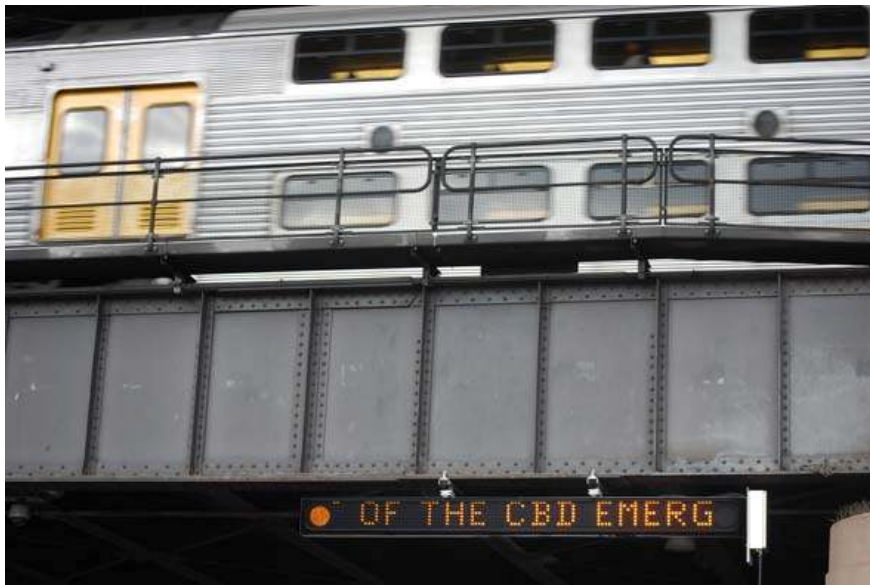
Figure 4 - Circular Quay Railway Station Variable Message Sign, radio/aerials
