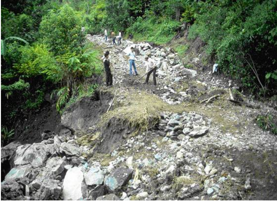
Figure 2 - A washed out rural road due to a plugged and overtopped culvert and lack of overflow protection.
