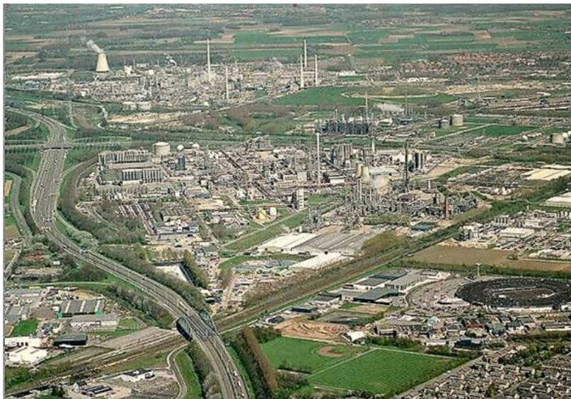
Figure 2 – Chemelot site (Netherlands)
