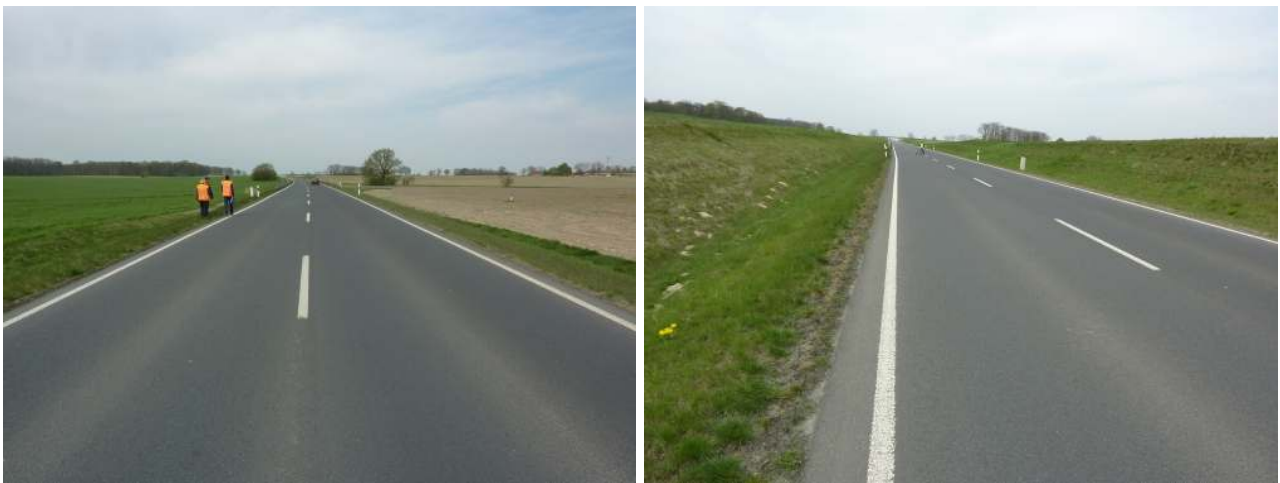
Figure 5 – View of embankment profile section (left) and cut profile section (right) in northerly direction
