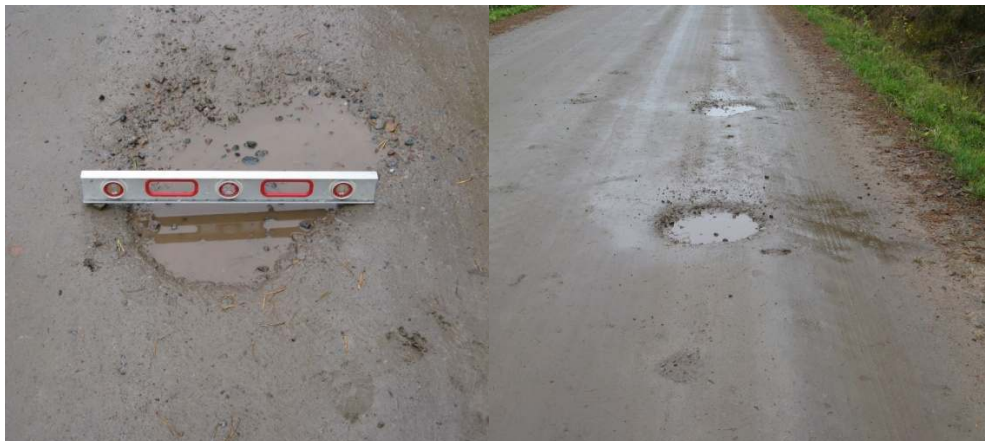
Figure 10. There were big depressions in the driving line of road 18613.
