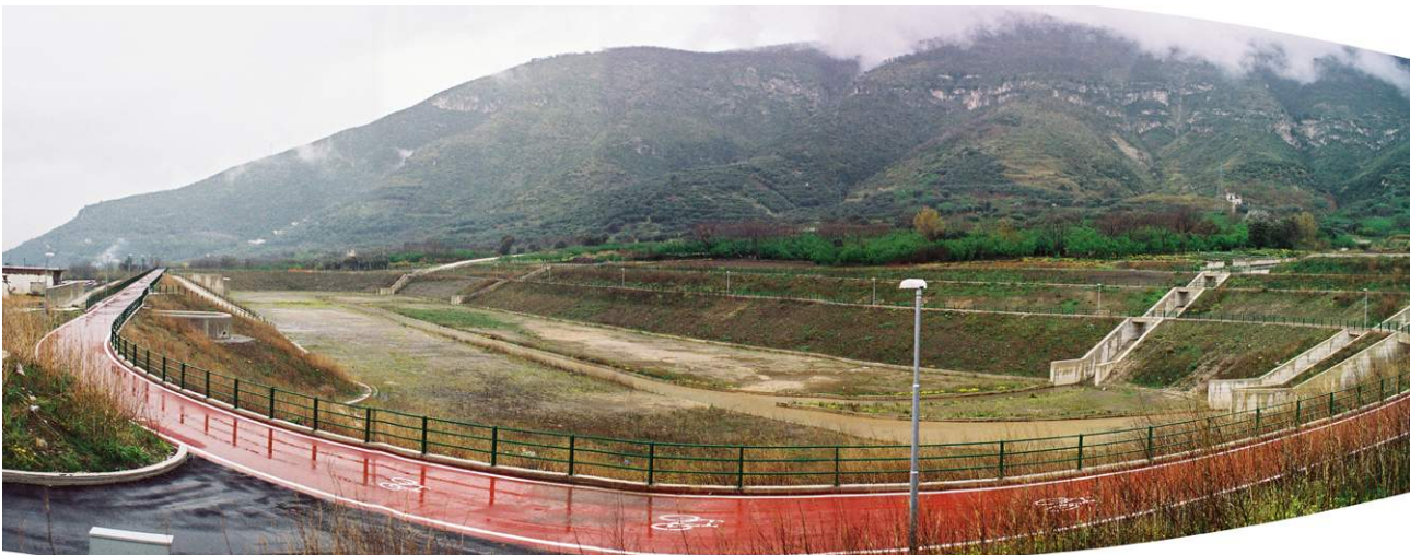
Figure 9 – Debris basin with a peripheral cycle track at Sarno in Italy.
