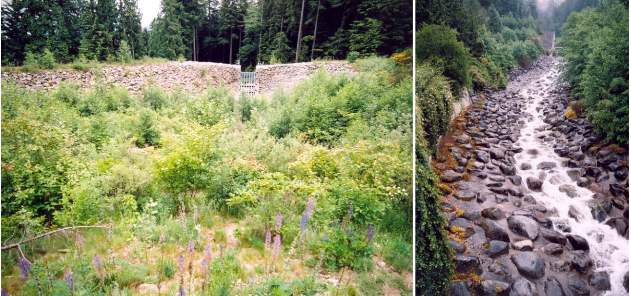
Figure 7 – Examples of a debris basin (left) and lined debris channel (right) from British Columbia in Canada.
