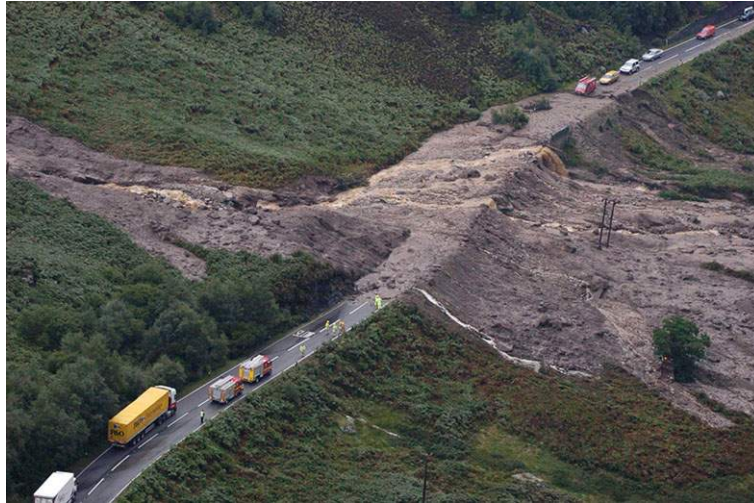
Figure 1 – Debris flow at A83 Glen Ogle on 18 August 2004.
