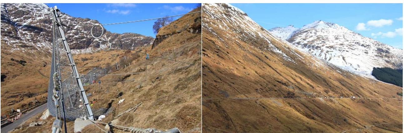
Figure 8 – A83 Rest and be Thankful debris fence: close-up (left) and distant views (right).
