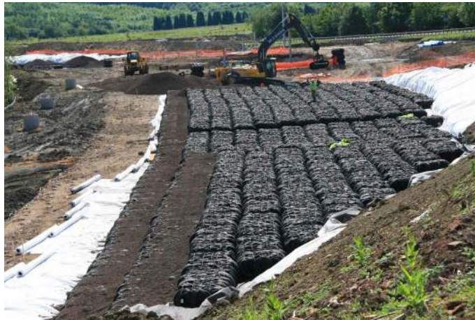
Figure 11 – Construction of the A421 embankment.
