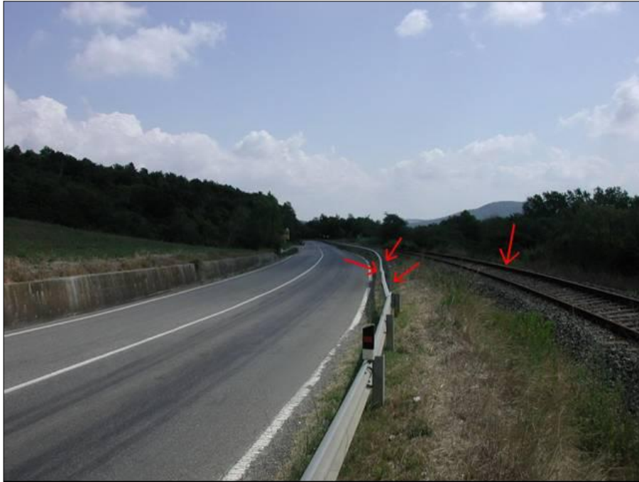
Figure 4 - Detachment from the posts, localised deformation, presence of the railway
