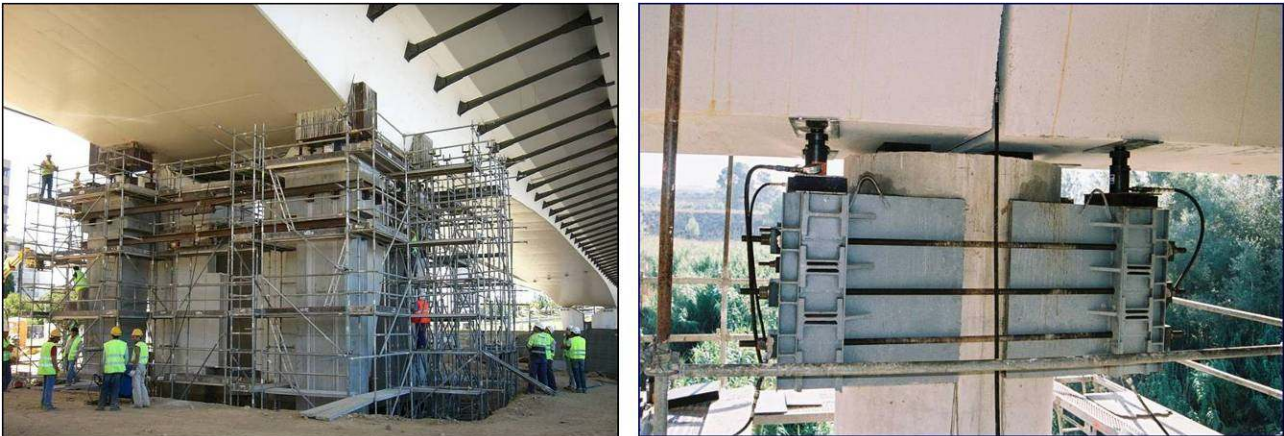
Figure 9. Example of action of maintenance specialized for the substitution of support equipment.
