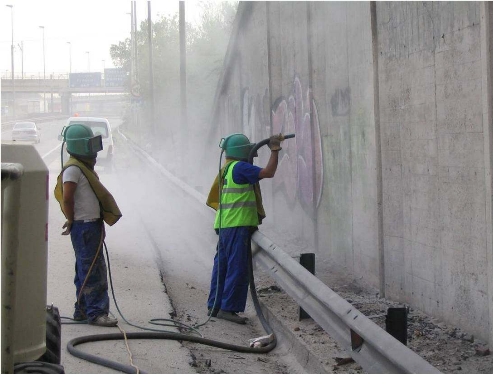
Figure 10. Example of action of ordinary maintenance of cleaning.
