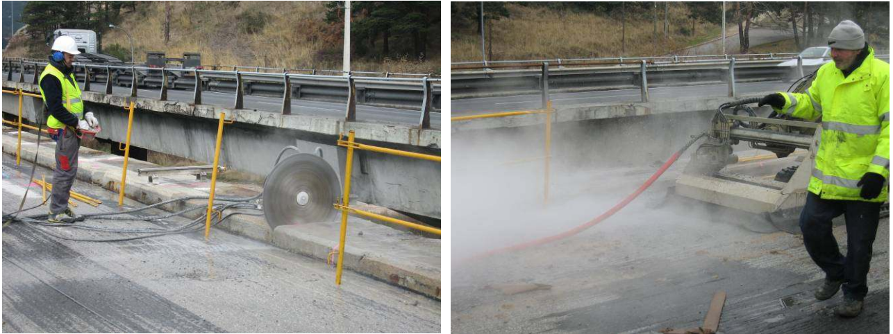
Figura 13 –Repairing works of the top slab of the deck of the Viaduct of San Rafael (AP-6)
