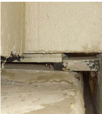
Figure 11 – An elastomeric bearing out of place, and a lack of cover of a prestressed tendon.
