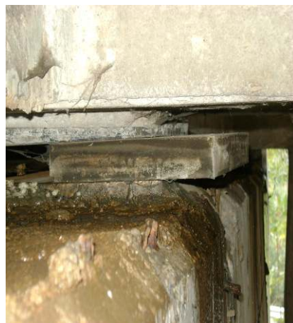
Figure 11 – An elastomeric bearing out of place, and a lack of cover of a prestressed tendon.
