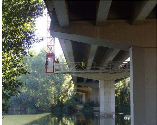
Figure 10 – General view of the self supported platform used for some inspections
