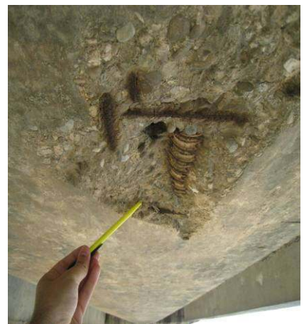
Figure 11 – An elastomeric bearing out of place, and a lack of cover of a prestressed tendon.
