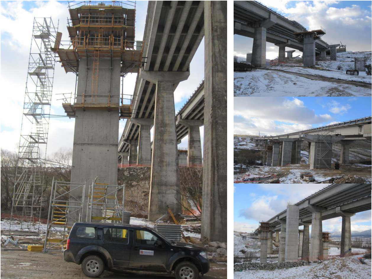
Figure 12 – General views of the repairing works of some bridges of the AP-6
