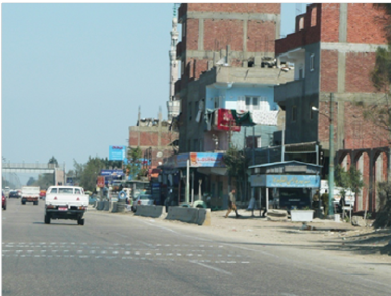
Figure 8: Example of a Motorway through urban areas without access control (Cairo-Alexandria Desert Road in Egypt)
