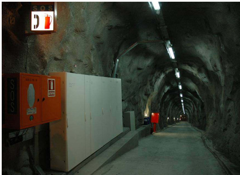
"Picture 6 – Inside the emergency passage"
