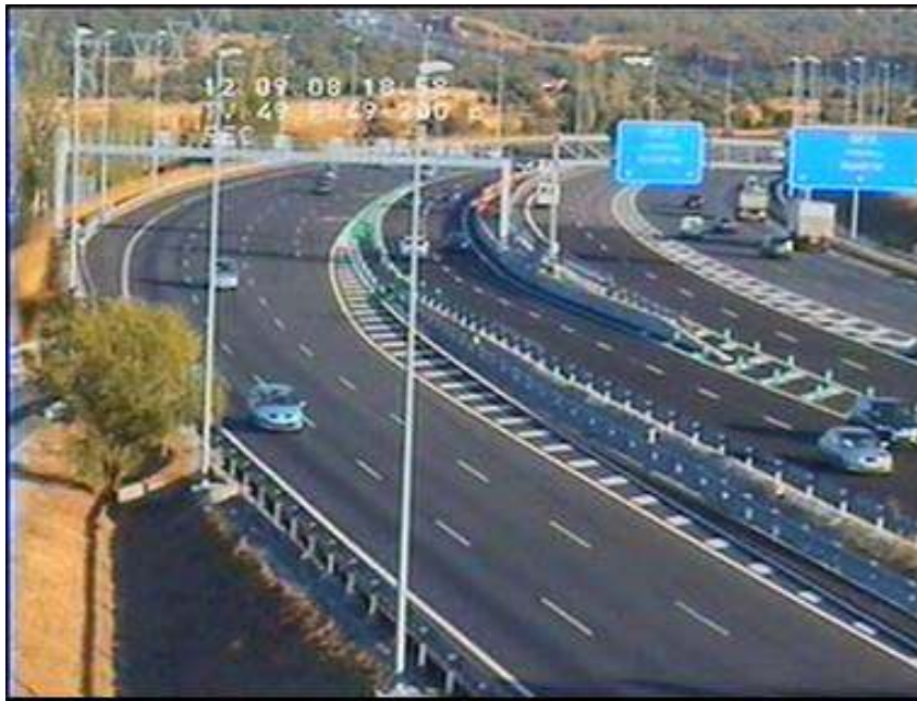
“Picture 1 – South Distributor”
