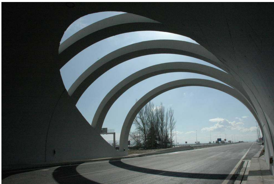
“Picture 7 – Exit tunnel 3”
