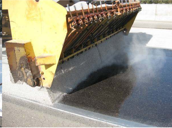
Figure 3: Machine application techniques used for SEAHC demonstrations.
