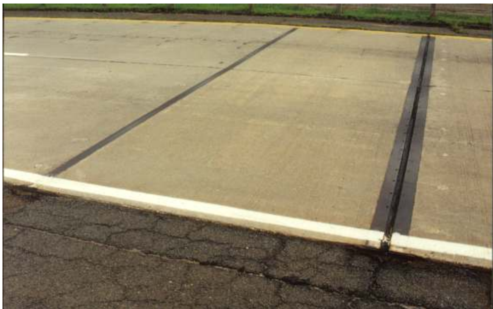
Figure 3 – Finished gap slab used in a PCP.
