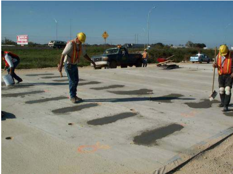
Figure 9 – Patching of central stressing pockets.
