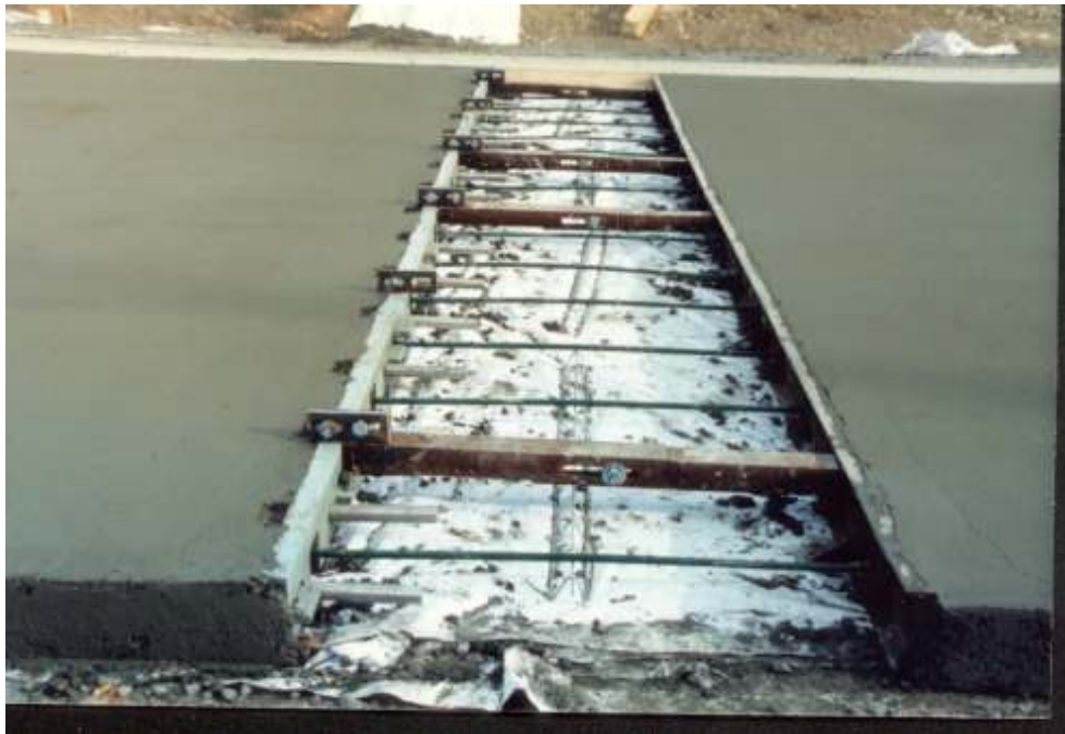
Figure 2 – Construction of a gap slab in a PCP.
