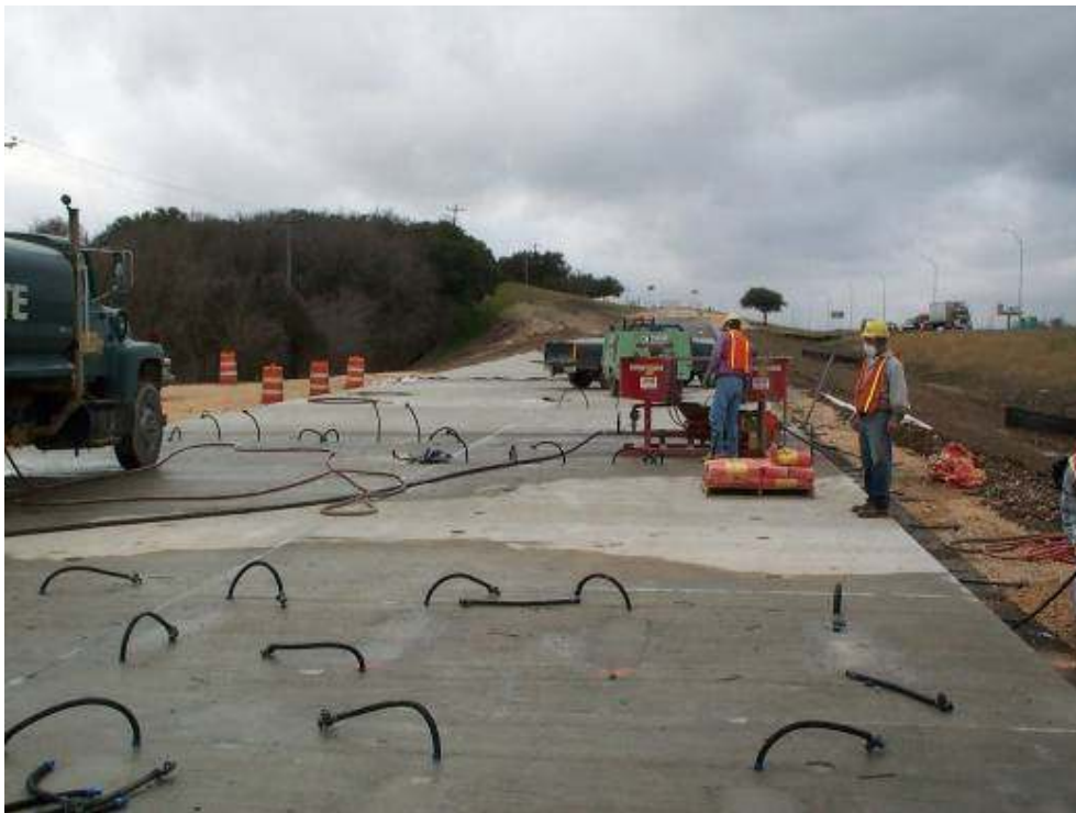
Figure 8 – Grouting operations after final prestressing stage.
