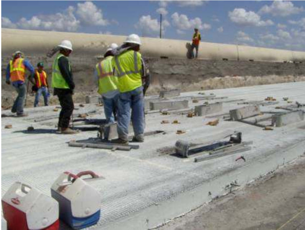
Figure 6 – Removal of steel forms from central stressing pockets.
