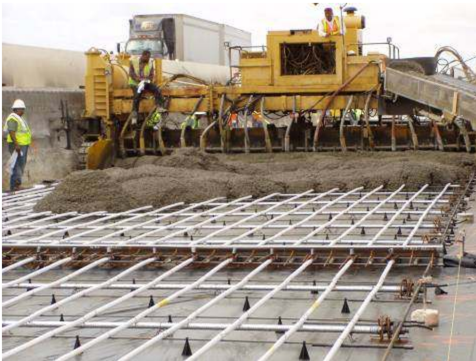
Figure 5 – Concrete paver and transverse joint of PCP.
