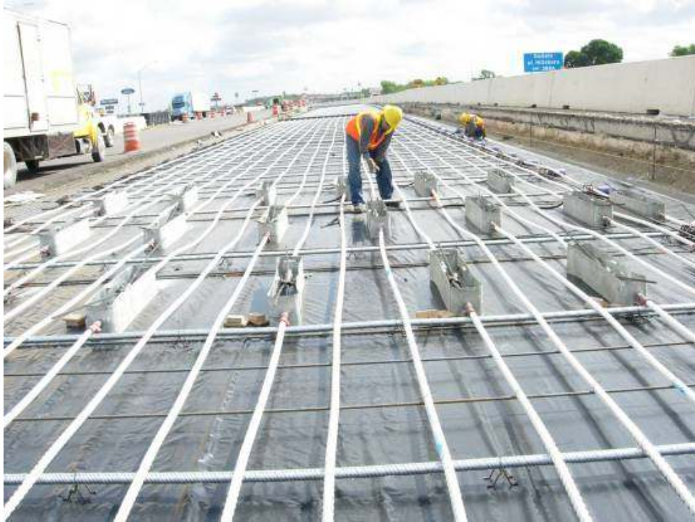
Figure 4 – Central stressing pockets used in a PCP.
