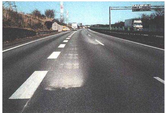
Photo 2 - Particles blowing up from Porosity
