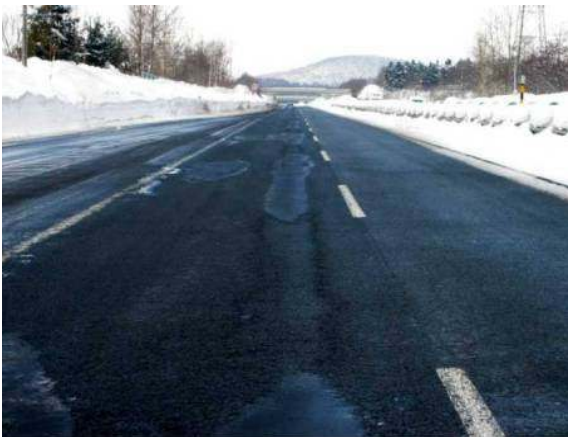
Photo 1 - Scaling and abrasion
