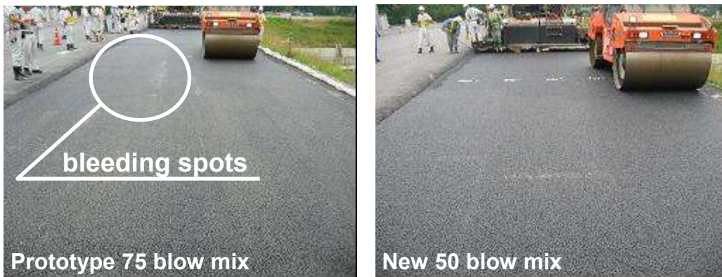
Photo 8 - Comparison of road surface [8]
