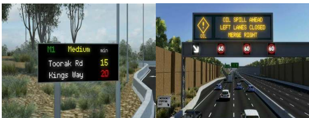
Figure 5 – VMS implemented on the M1 Freeway
