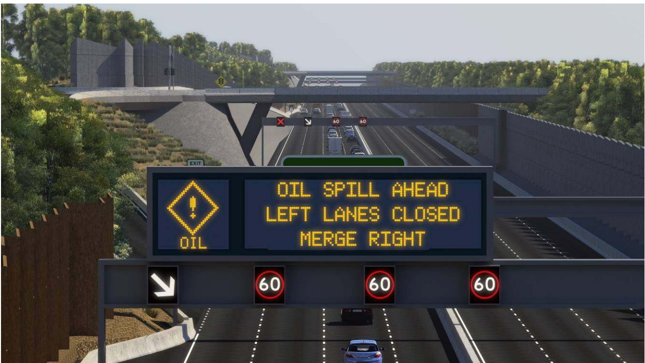
Figure 2 – Lane Use Management (LUM) and Variable Message Sign (VMS)
