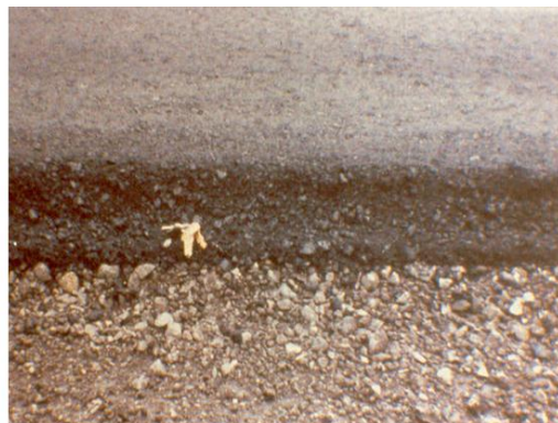
Figure 11 - Mixing and compaction of sub-base (25 cm) and base courses (20 cm). Crushed gravel. Puebla - Orizaba highway
