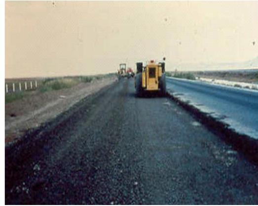
Figure 9 - Mixing and compaction of sub-base (25 cm) and base courses (20 cm). Crushed gravel. Puebla - Orizaba highway
