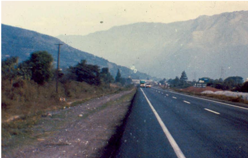
Figure 13 - Completed “Inverted section” pavement. Mexico – Puebla highway
