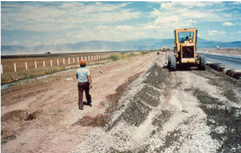
Figure 8 - Mixing CCR elements of figure 7. Guadalajara - Colima highway
