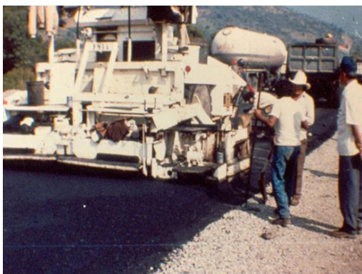
Figure 11 - Mixing and compaction of sub-base (25 cm) and base courses (20 cm). Crushed gravel. Puebla - Orizaba highway
