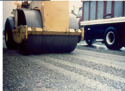
Figure 10 - Surface course of asphalt concrete (10 cm). Guadalajara - Colima highway
