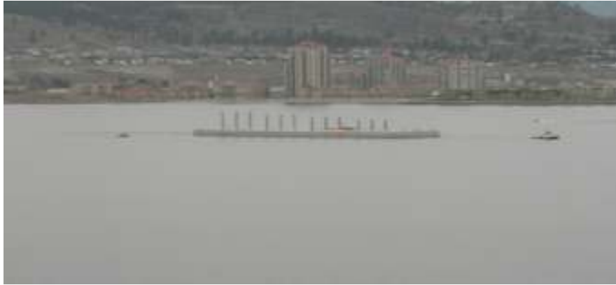
Figure 6 – Towing the pontoons to the bridge site
