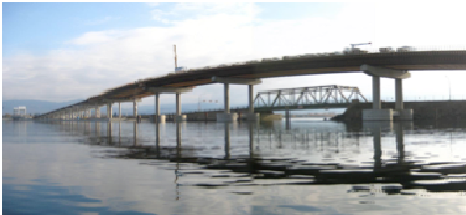
Figure 5 - The fixed elevated span and the navigation channel
