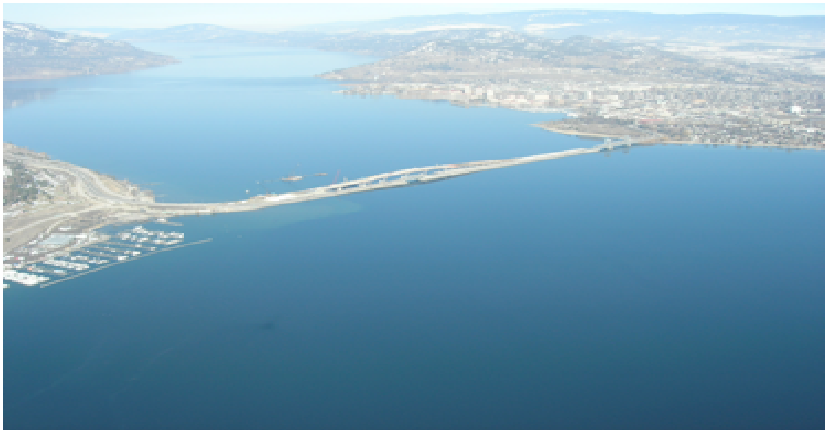
Figure 8 – Closing the gap for the new bridge
