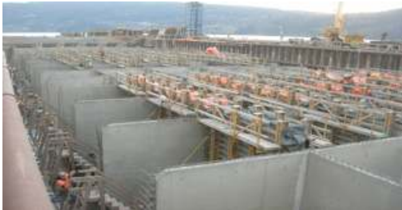
Figure 4 – Fabricating the pontoons
