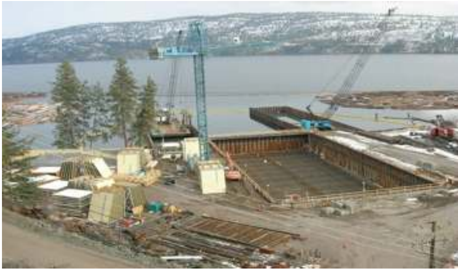
Figure 3 – Constructing the Graving Dock
