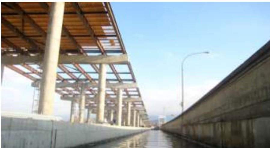
Figure 7 – Constructing the floating elevated section
