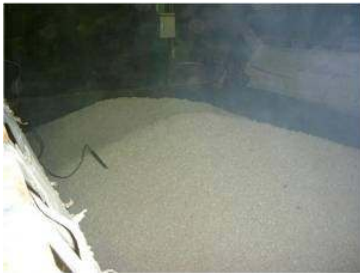
Photo 7 - Mixing and laying CERAM
