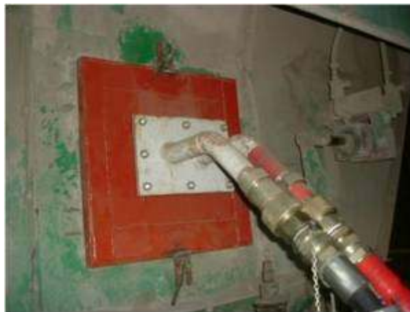
Photo 5 - Inlet of epoxy resin
