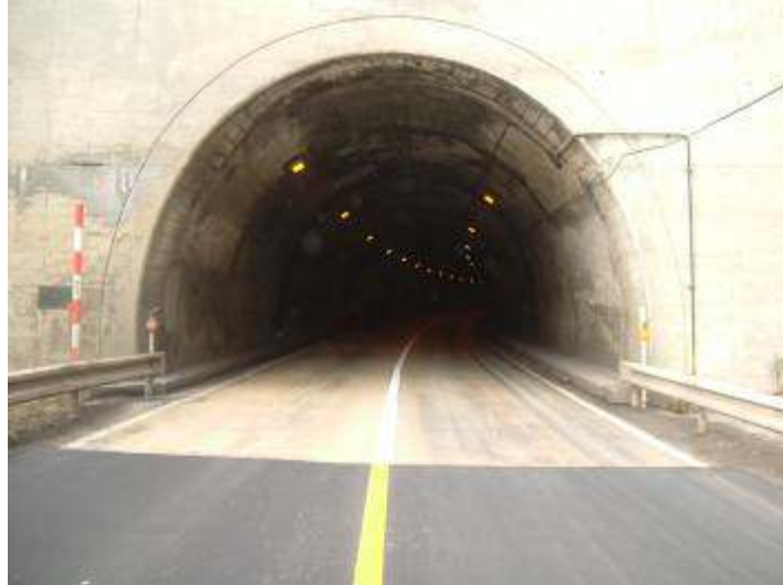
Photo 9 - Completed CERAM pavement
