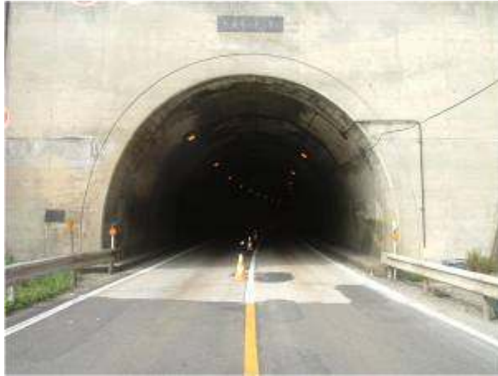
Photo 6 - Tunnel of CERAM construction (before CERAM construction)
