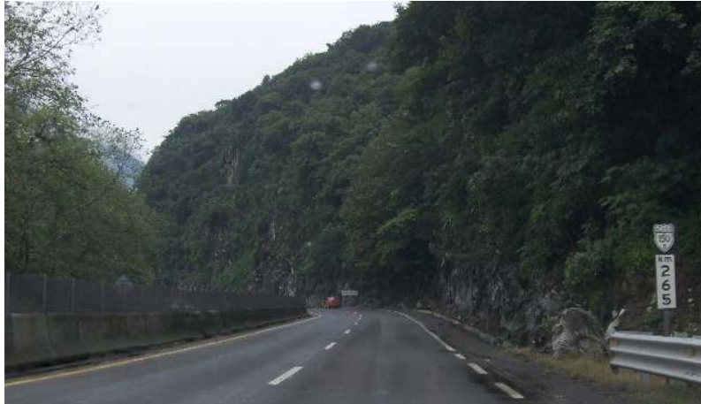
FIGURE 4 Cut slope at Segment 3
