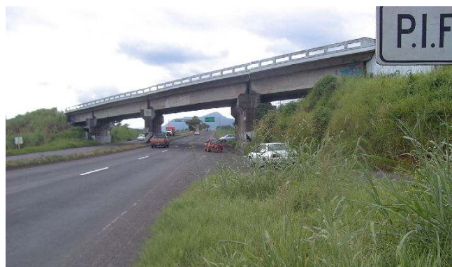
FIGURE 11 Conditions of the incorporation into the expressway at Segment 10
