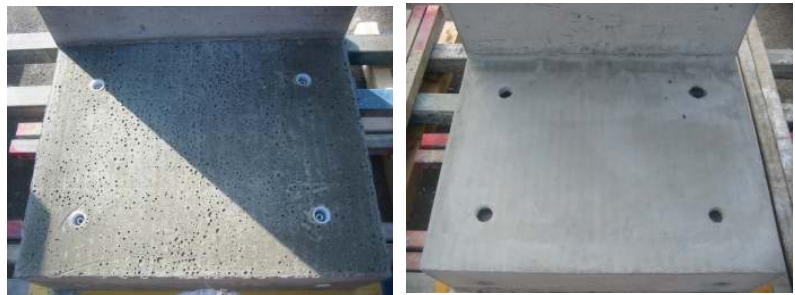
Photo 2 - Improvement of finished concrete
