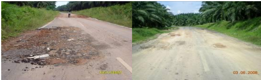
Figure 8 - Pavement defects
