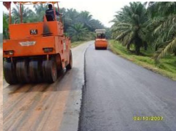
Figure 6 - Compaction of ACWC
