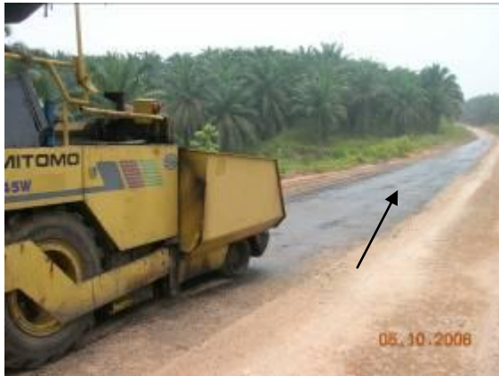
Figure 5 - Prime coating
