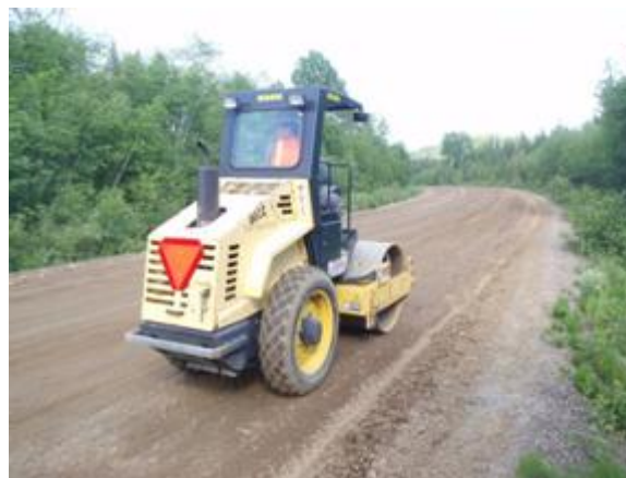
Figure 7 – Roller compactor used for compaction of the control and stabilized section
