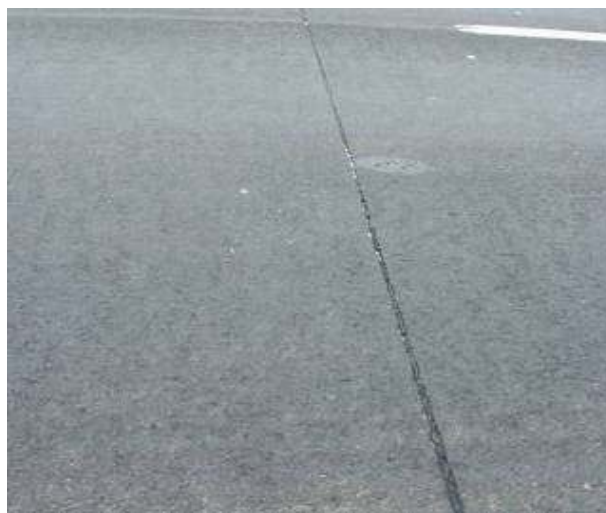
FIGURE 14. Micro-surfacing over a concrete pavement.
