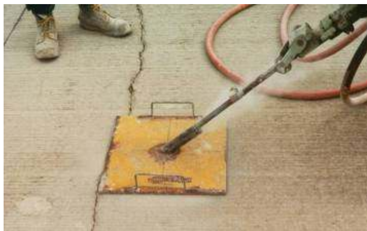
FIGURE 2. Drilling holes for cross stitching.
