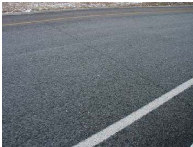
FIGURE 15. Thin asphalt concrete overlay over a concrete pavement.
