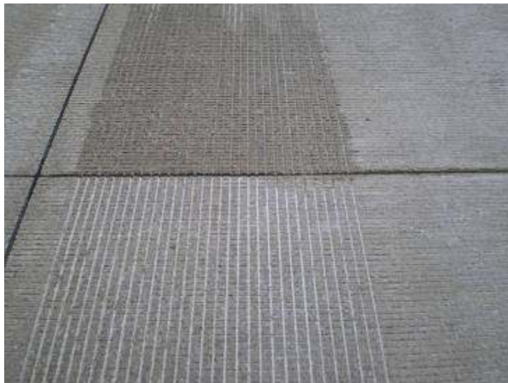
FIGURE 10. Longitudinal grooving completed perpendicular to the transverse tines.
