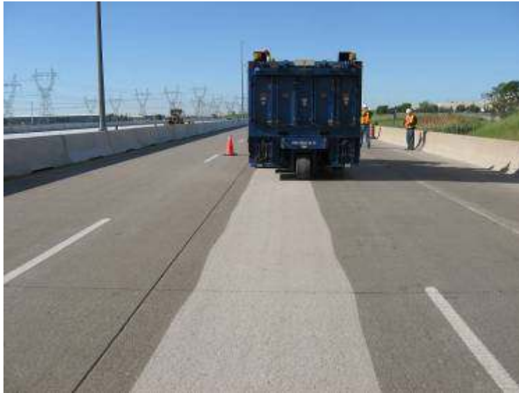
FIGURE 11. Blastrac concrete pavement surface texturization.
