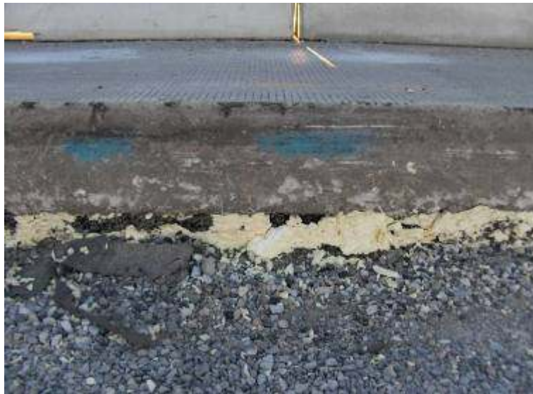
FIGURE 12 Slab jacking using foam.
