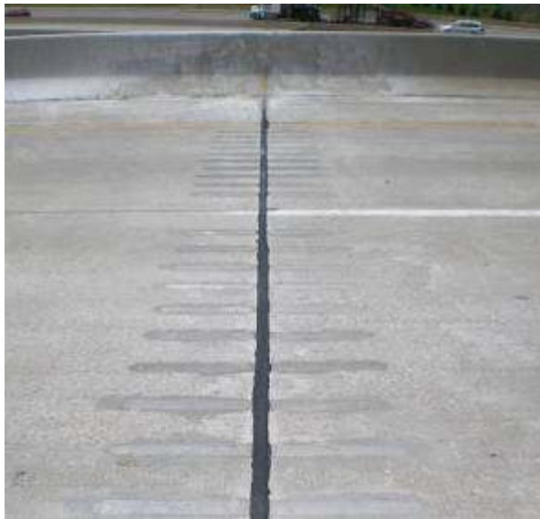
FIGURE 8. Expansion joint retrofit at bridge approach.
