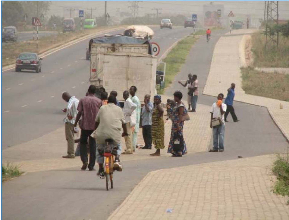
Figure 13- Segregated road way, cycle lane, pedestrian walkway on the N4
