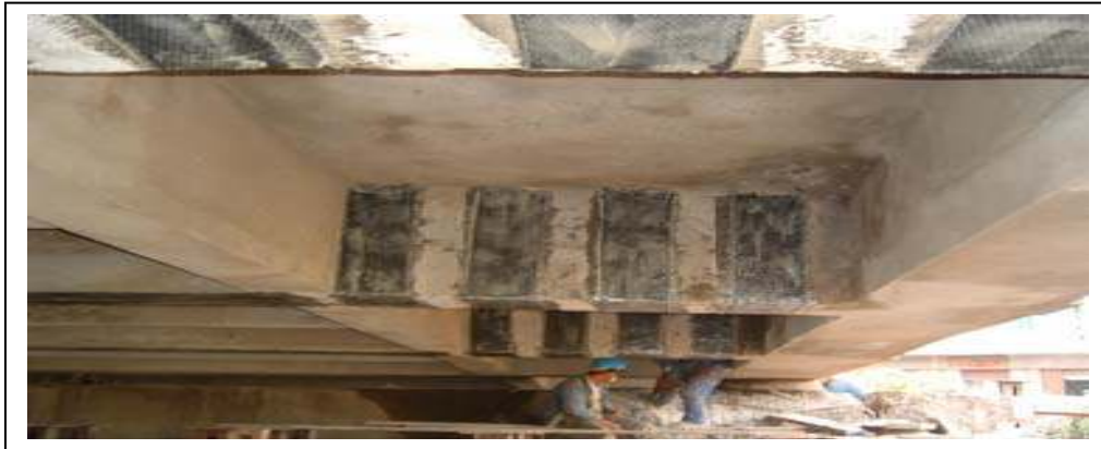
Figure 5 - Application des composites CFRP
