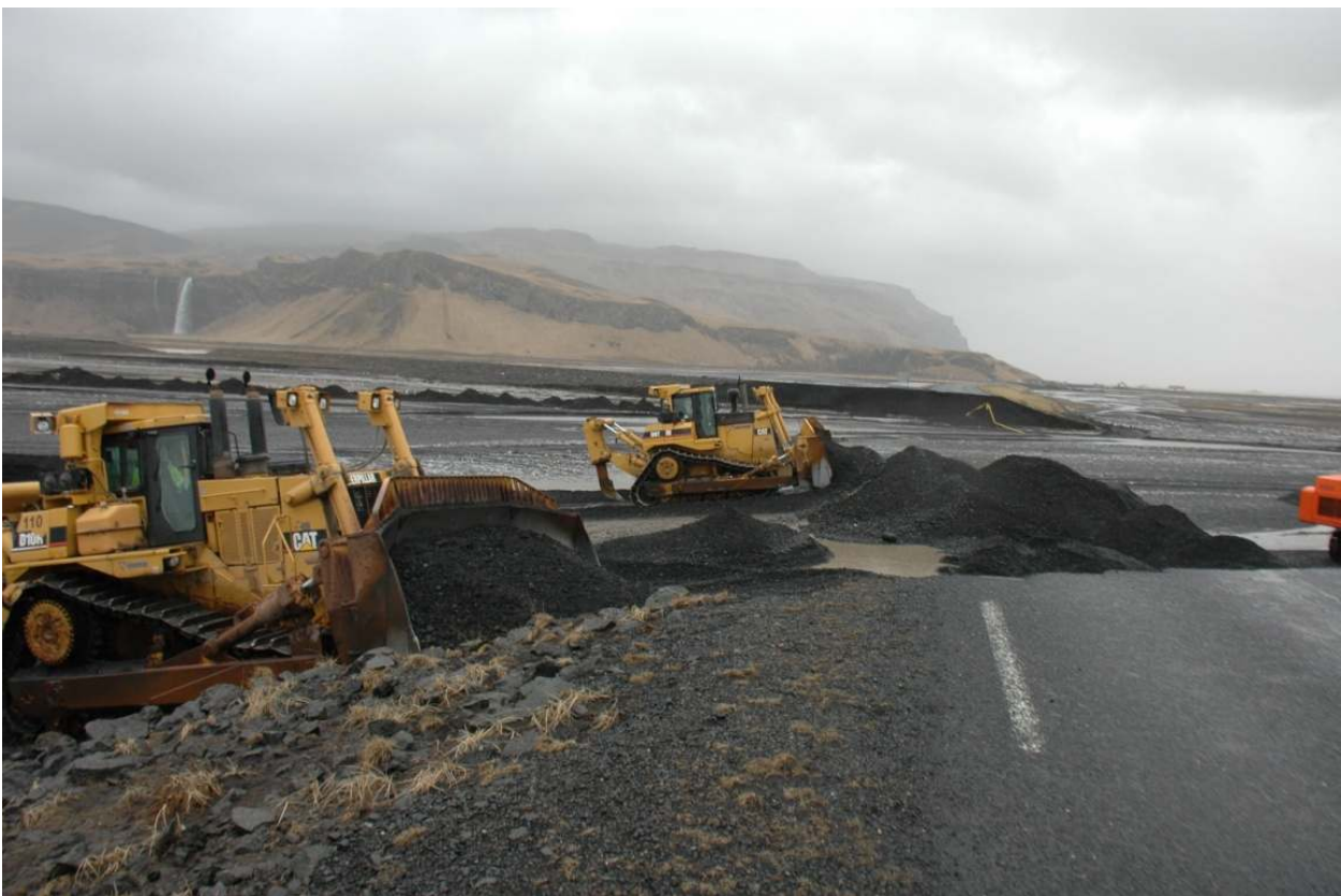
Figure 11 – Rebuilding of roads started already the day after the catastrophic flood.
