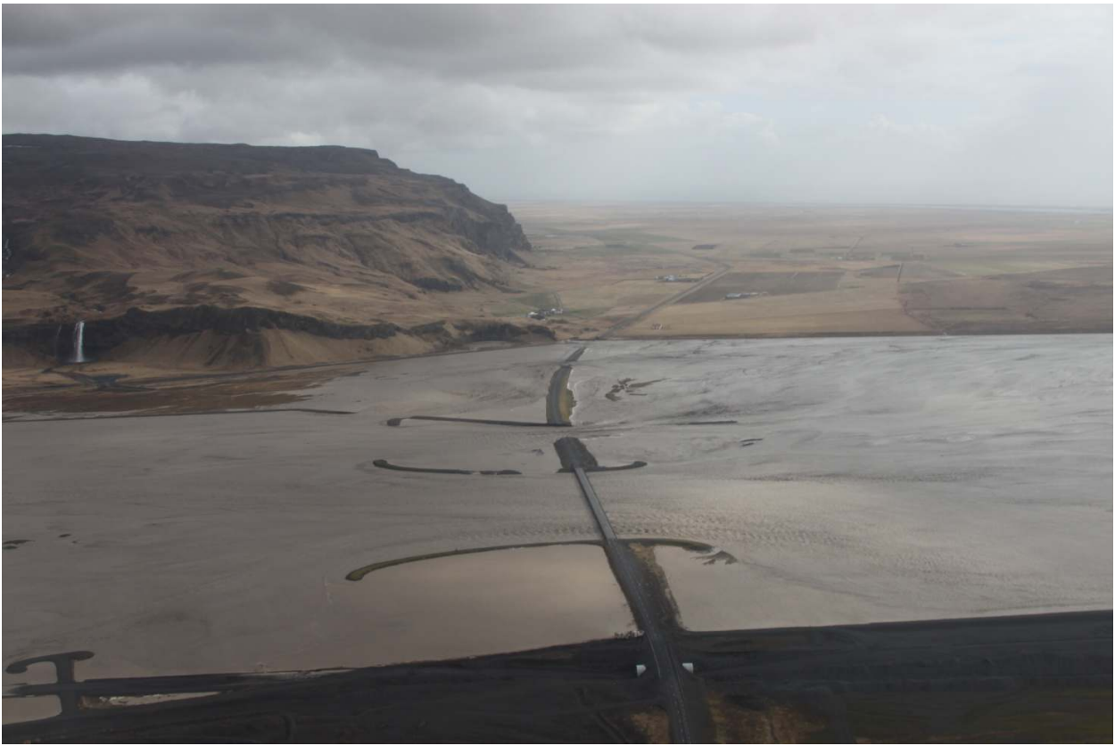
Figure 10 – The flood at maximum discharge at Route 1. Roads and dams were damaged.
